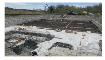
By using Xypex Admix C-500, the reservoir achieved integral waterproofing without relying on external membranes or coatings, simplifying construction while providing a barrier against water ingress. The use of Xypex Admix C-500 also enhanced the concrete's resistance to chemical attacks and significantly reduced future maintenance costs.
